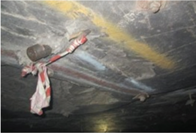
Borehole entering the hanging wall
