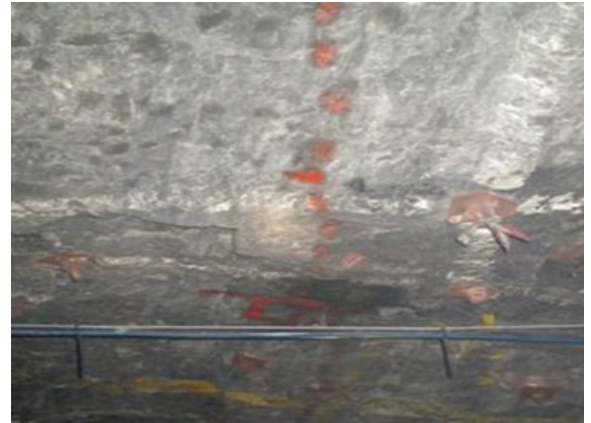
Cabling encountered along survey line
