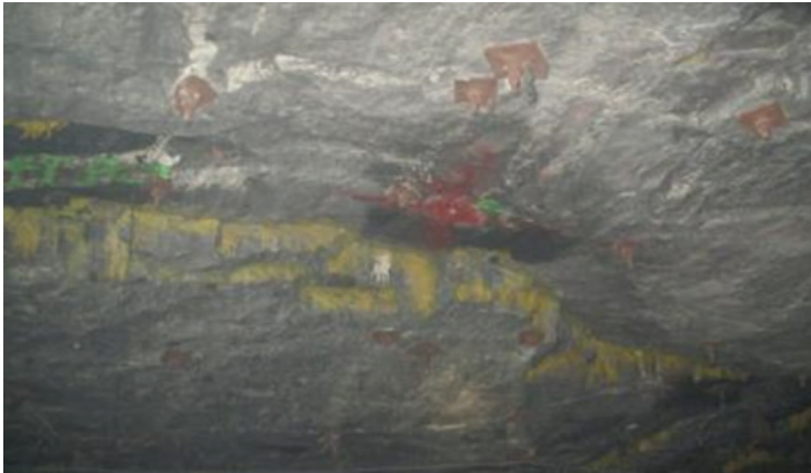
Sharp brows and bolts encountered along survey line
