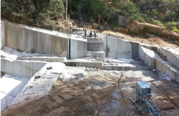
Overview of quarry site
